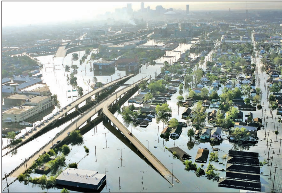
Floodwaters from Hurricane Katrina fill the streets near downtown New Orleans in this Aug. 30, 2005, file photo. Despite billions of dollars in aid, recovery programs with catchy names and an outpouring of volunteer effort, two years later, much of New Orleans has still yet to recover from the fury of the storm. (AP photo/David J. Phillip, file)
